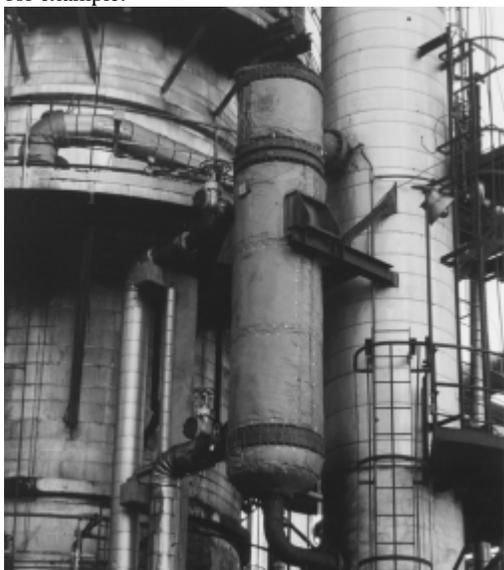
Figure 1 – Reboiler Heat Exchanger
